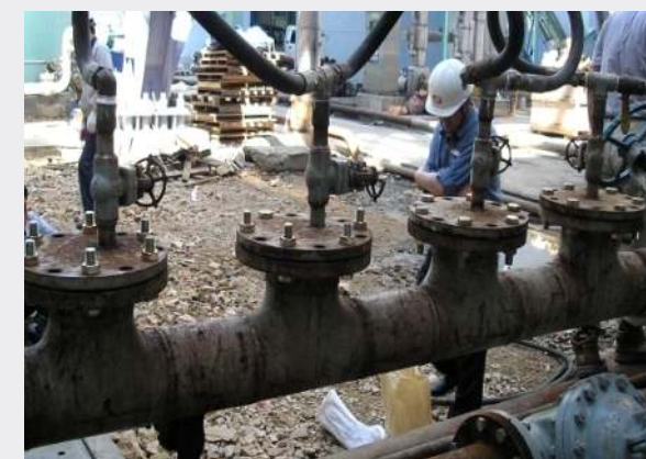
Test Coupon설치
