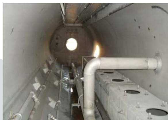
After Chemical Cleaning
